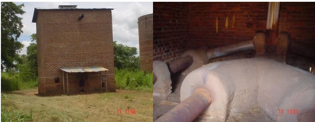
Figure 3: External and internal view of Convention Barn
