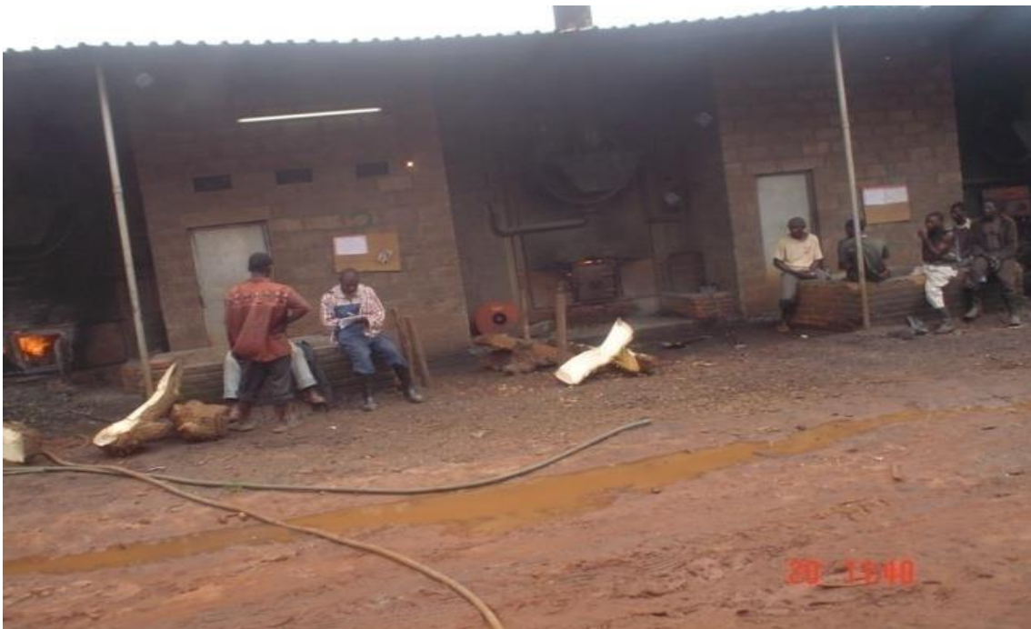
Figure 8: External view Tunnel Barn with the furnace,
