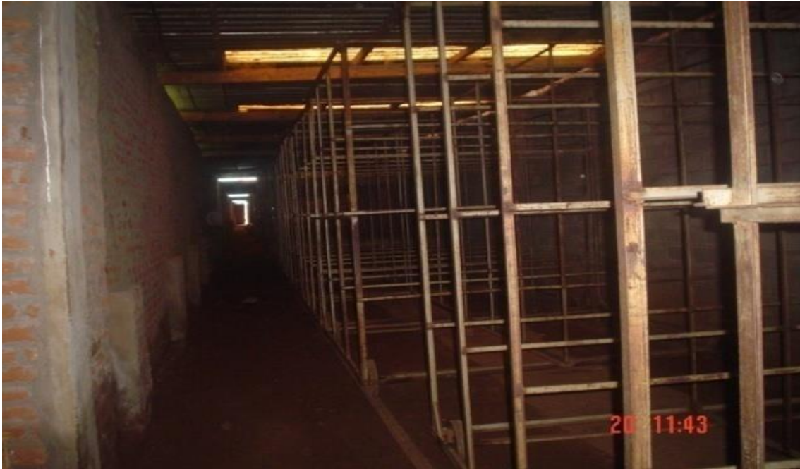
Figure 7: Internal view of a tunnel barn and trolleys in their rails ready to hang the leaves
